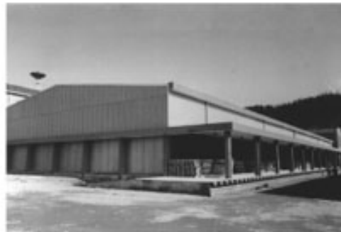
Shandong Peanut Warehouse, Shandong, PRC 28 x 85 x 5 m. 8 compartment
